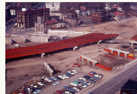
I-81 corridor construction
